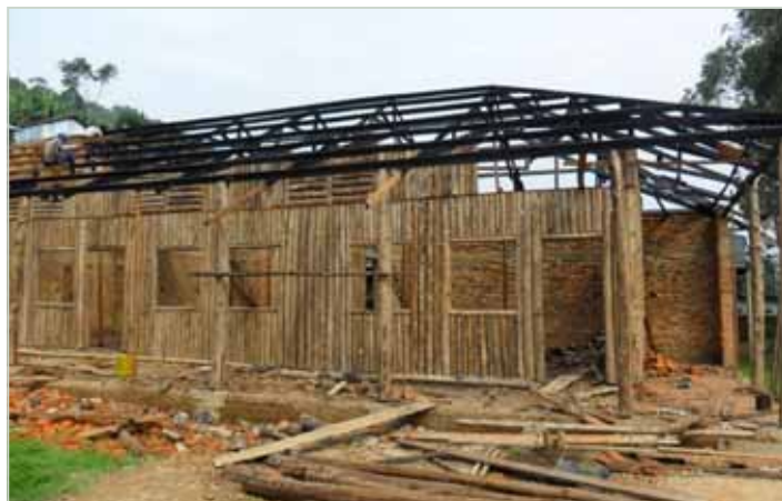
Batwa Women's Center nearing completion
