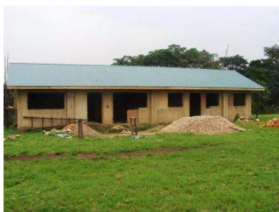
Trade school at Byumba nearing completion
